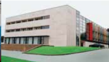
The Mogosoia centre and stadium.
